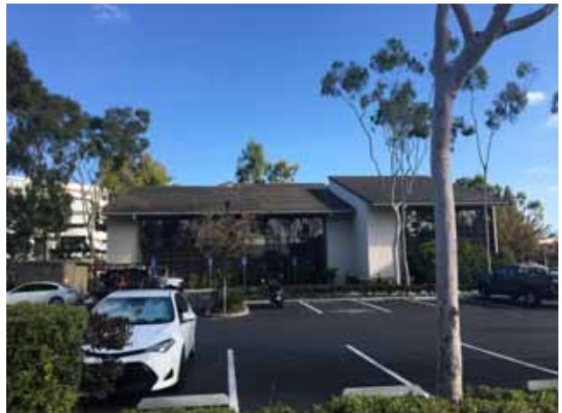
24. View of the north adjacent property
