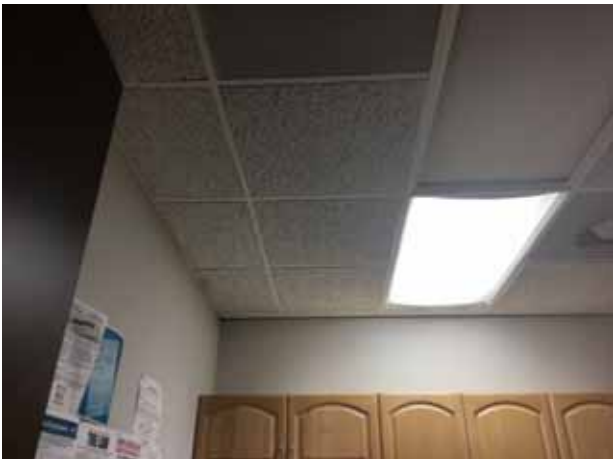
17. View of the subject property: ceilings
