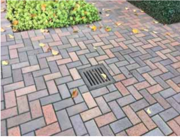
7. View of the subject property: storm drain
