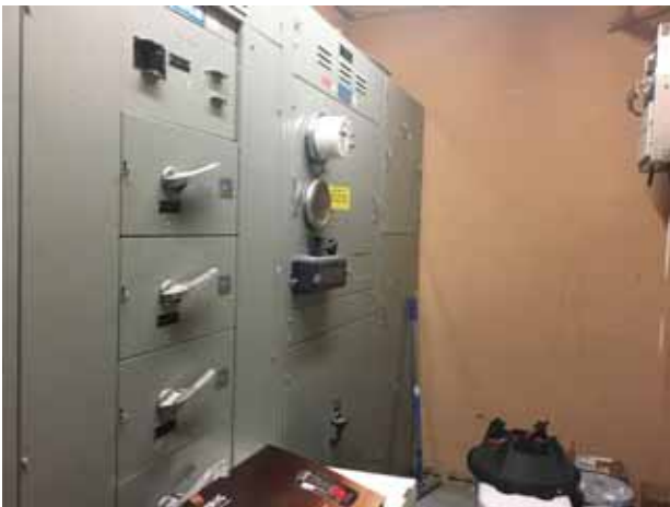
15. View of the subject property: electrical panel
