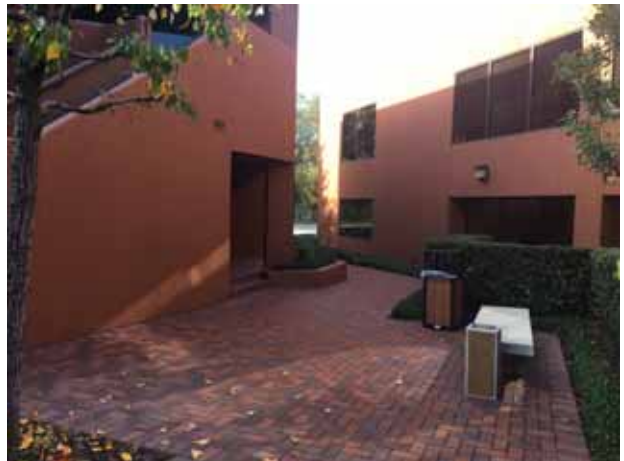
6. View of the subject property: patio area
