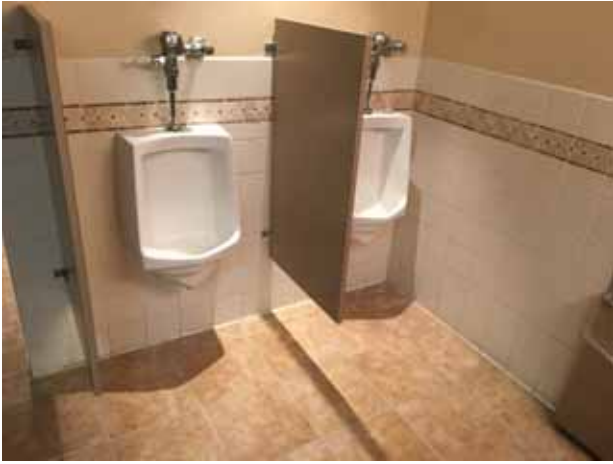
19. View of the subject property: bathroom
