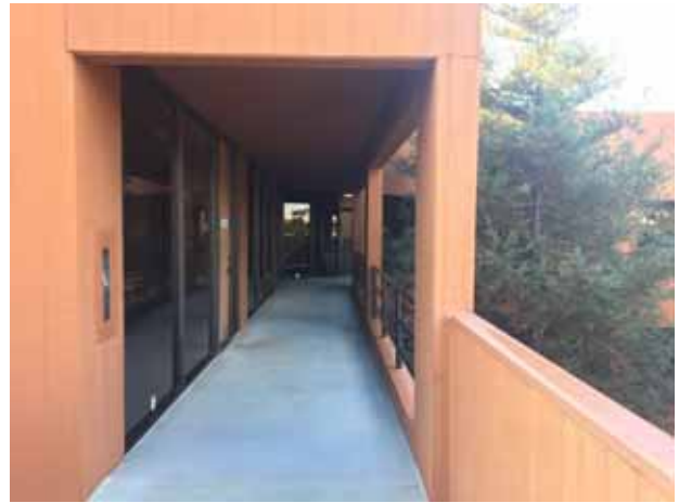
10. View of the subject property: balcony
